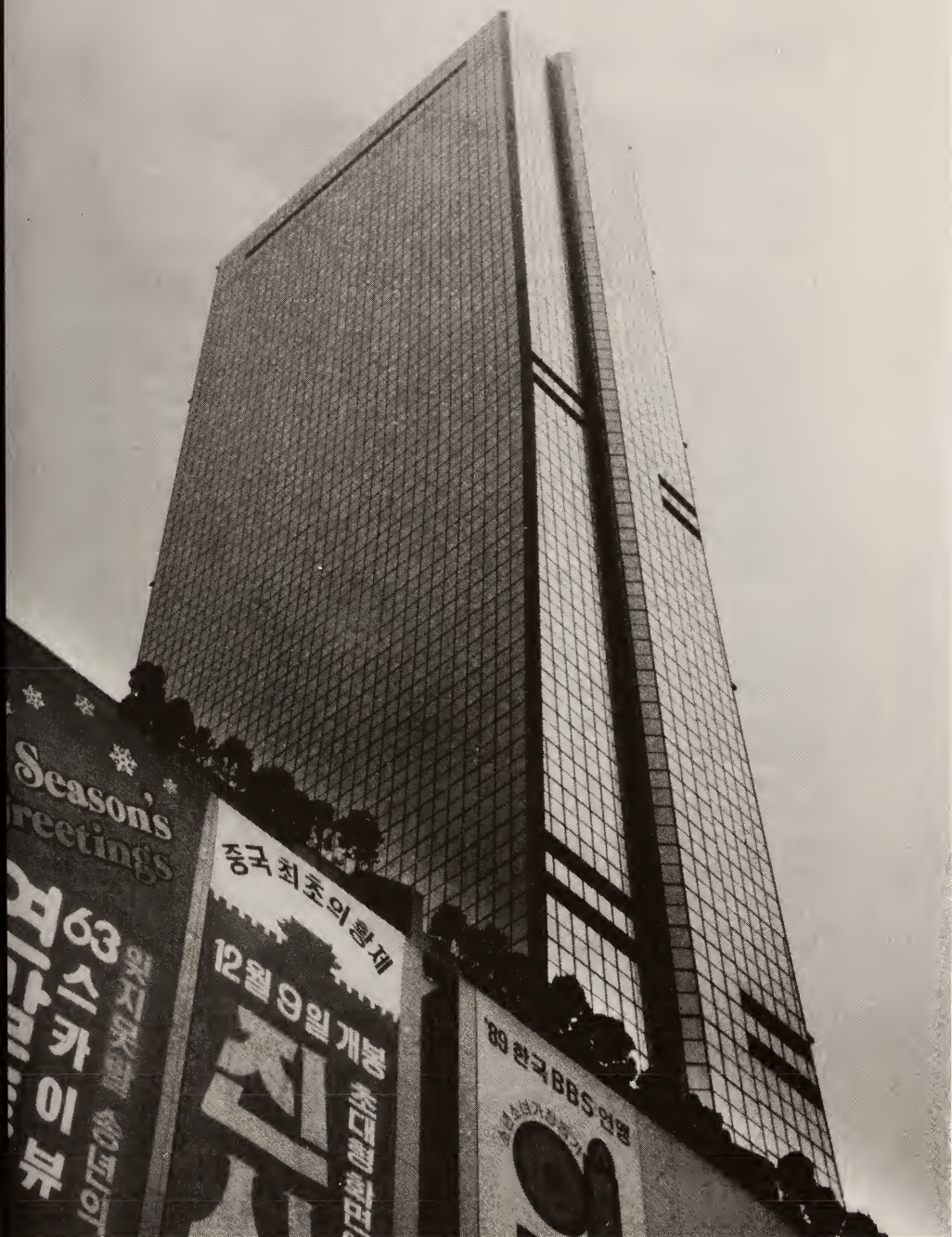
Sixty-three-story Daehan Life Insurance Building, a popular tourist attraction and one of the tallest buildings in Asia Courtesy Oren Hadar
